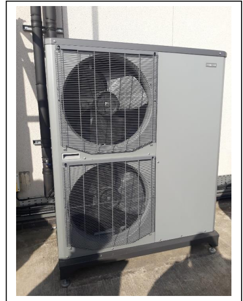
Figure 8: Air Source Heat Pump: AAC Flintshire Dobshell
