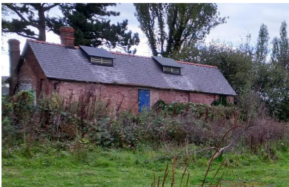
Bat Roost at Flintshire MRD
