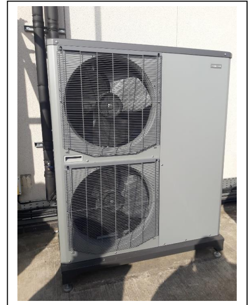
Figure 8: Air Source Heat Pump: AAC Flintshire Dobshell
