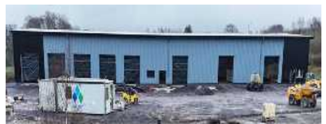
Photo 2: Bangor Fleet Workshop (under construction)
