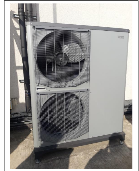
Figure 8: Air Source Heat Pump: AAC Flintshire Dobshell
